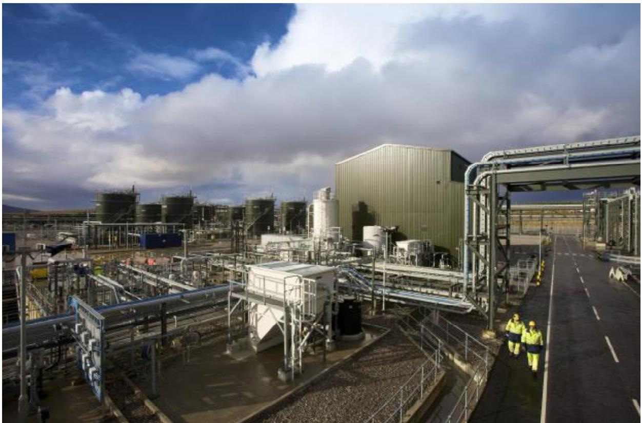
Esmil Process Systems Ltd, one of the UK's leading experts in the field of oil water separation and treatment have recently completed a large RWWTP (Refinery Waste Water Treatment Package) for the Corrib project in Ireland on behalf of Shell and AMEC.
