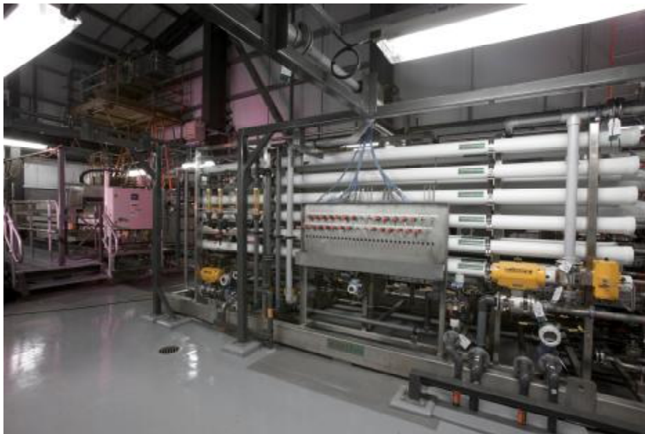
Membrane Skid for Ultra-filtration Membranes
